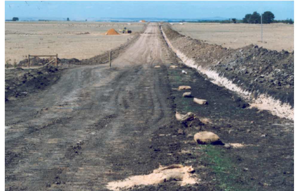
Contrasting shallow black self mulching soils on the rise and grey soils on the lower plain
